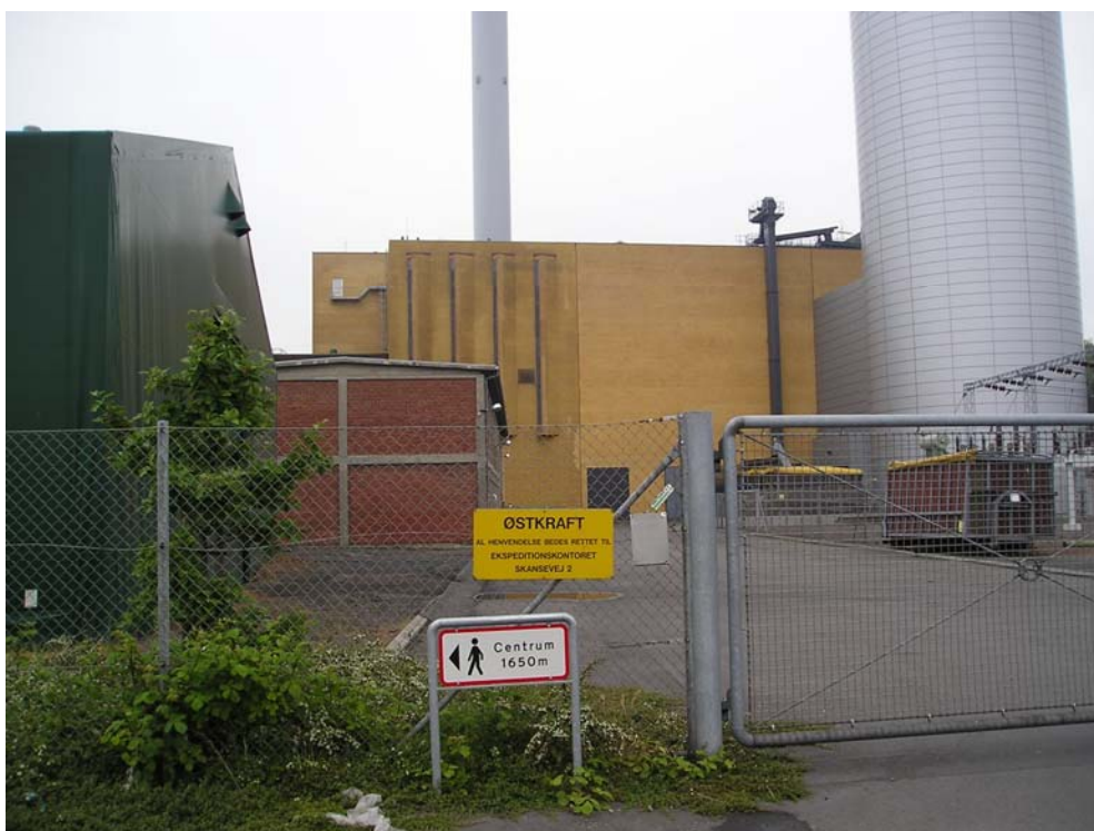
Figure 4. Port of Rønne, industrial environment
